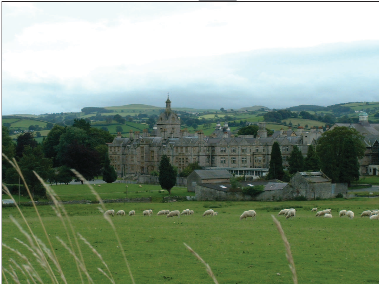
Picture 2: View towards the site from crossroad of B4501 and Ystrad Road
